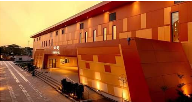
Exhibition Hall (Vayu Hall), Advanced Training Institute (ATI), ONGC, Goa, India
