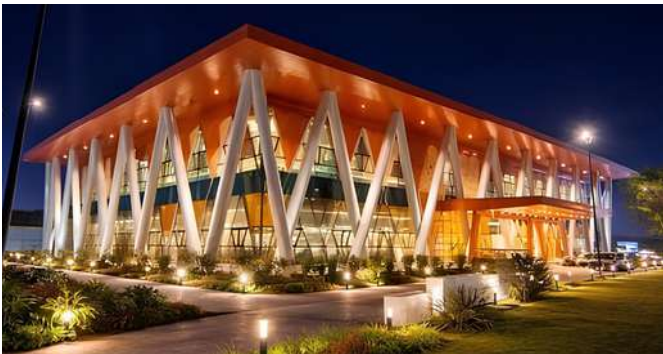
Management Development Facility (Akash Hall), Advanced Training Institute (ATI), ONGC, Goa, India
